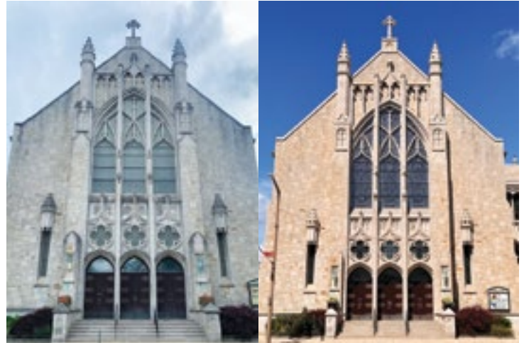
First United Methodist Church before and after renovation
